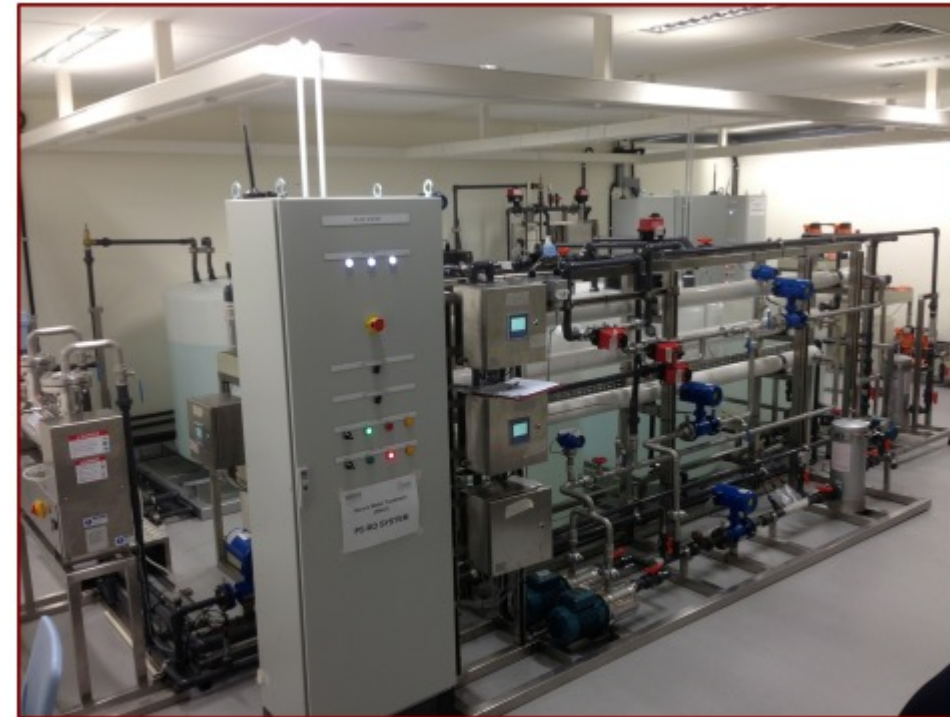
Fig. 1: Actual Photograph of SWaT testbed
