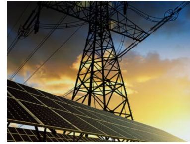
Power System Controls
